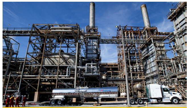
The Shell Norco Manufacturing Complex in the USA uses liquid feedstock made from plastic waste to make chemicals.
