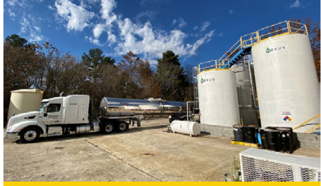
Shell and Nexus Fuels LLC have a supply agreement for pyrolysis liquid made from plastic waste, which is then converted into chemical products.
