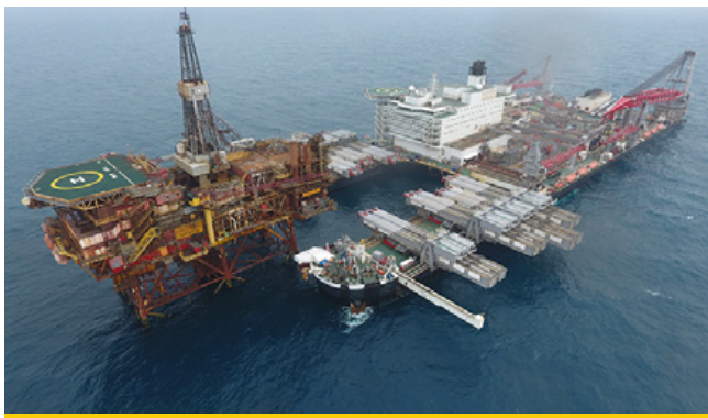
The Pioneer Spirit vessel removed the part of Brent Alpha visible above the sea in a huge single lift.
