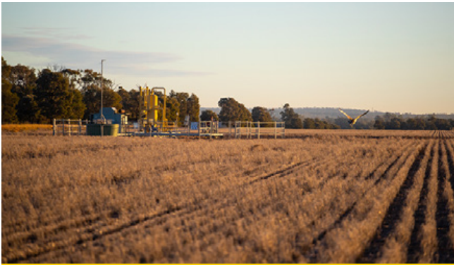
The Shell-operated QGC natural gas wells in Queensland, Australia, where sustainability considerations include endangered ecosystems and essential habitats.
