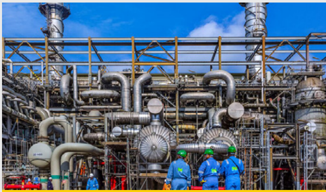
The Nigeria LNG joint venture's expansion project is expected to create about 12,000 direct jobs during construction.
